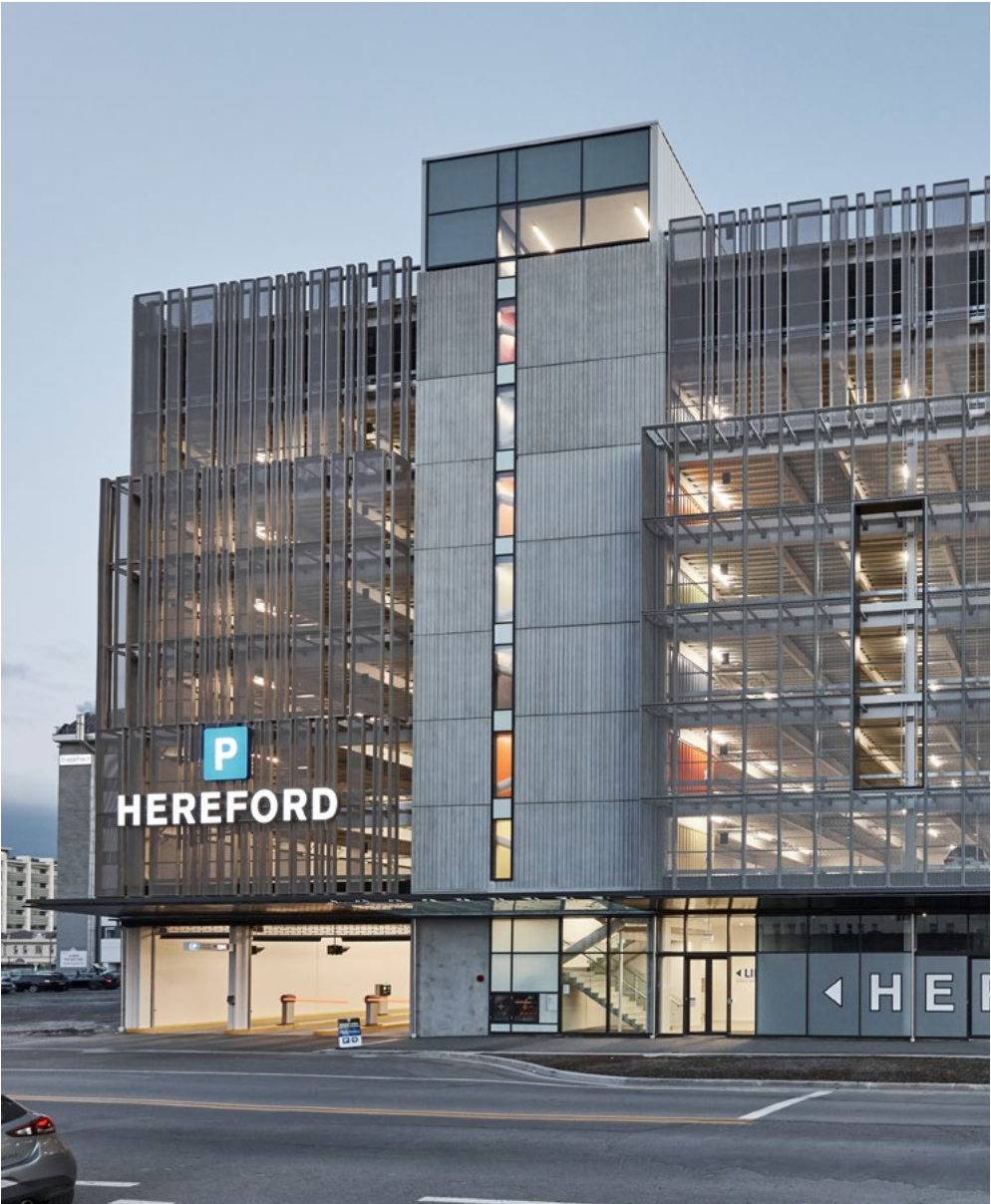
Hereford Street Car Park, Christchurch | Custom Mesh
