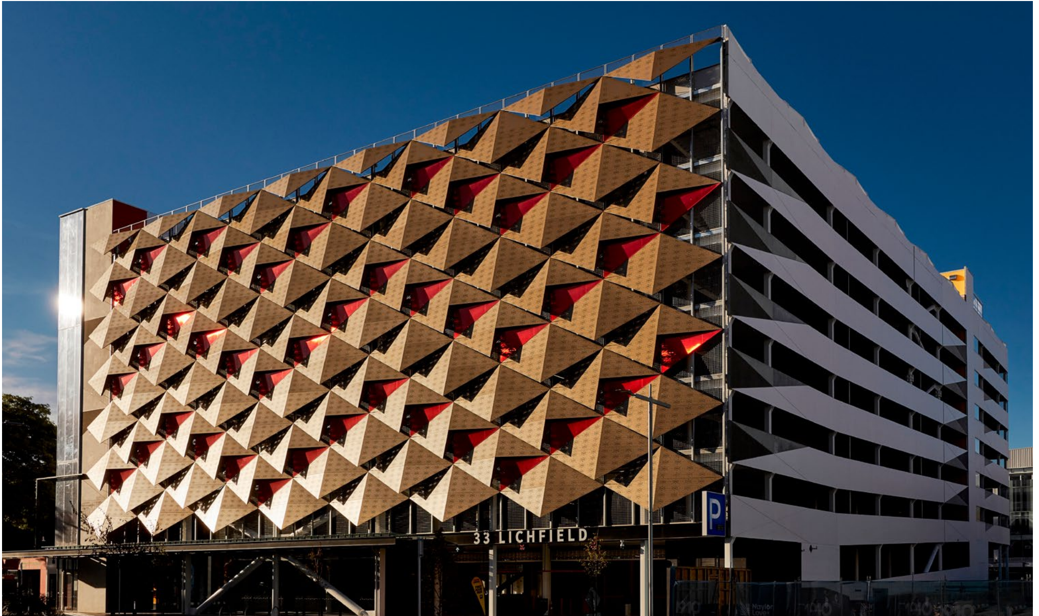
Lichfield Street Car Park, Christchurch | Custom Dapple
