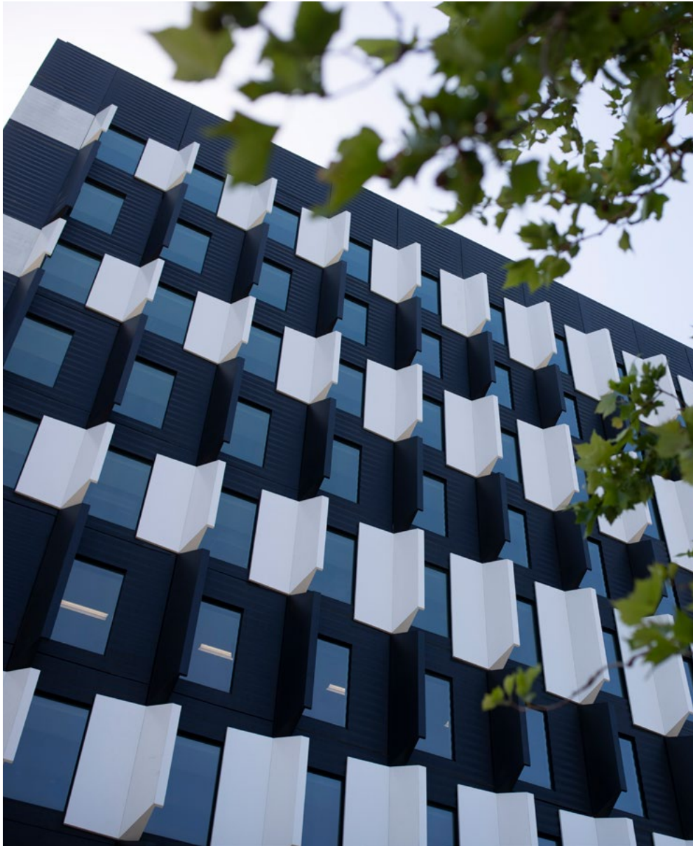
Sylvia Park Tower, Auckland | Custom Sunshade Fins and Vertical Louvres
